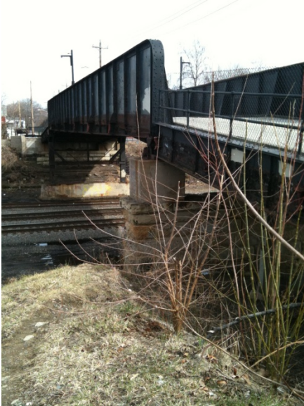
15 th Street Bridge Looking East
