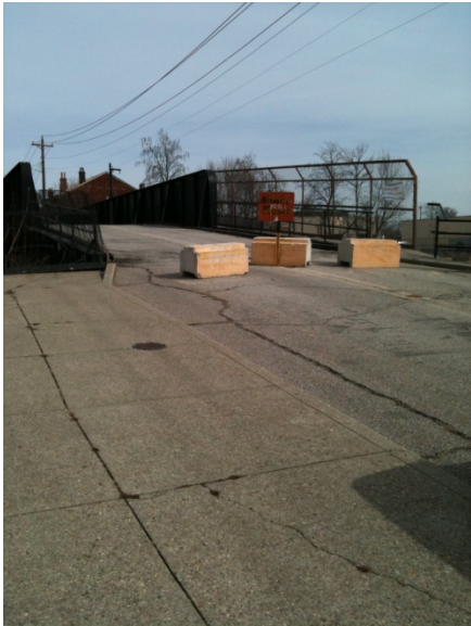
15 th Street Bridge Looking East
